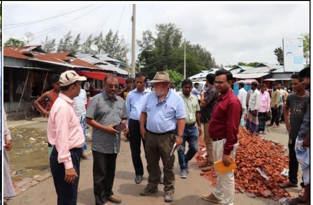
IFAD and EKN mission members visit road construction works
