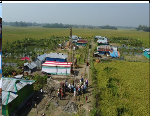
Support for Hand DTW sinking for RAP family
